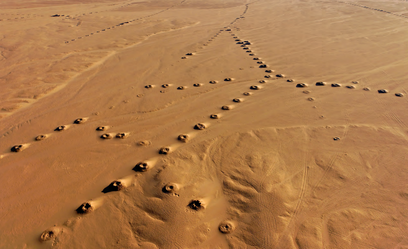
Parts of Akabli's qanat system, above, has had no maintenance for some three decades, yet it continues to provide ample water to local gardens, lower, where a farmer controls his irrigation by opening and closing small channels.
