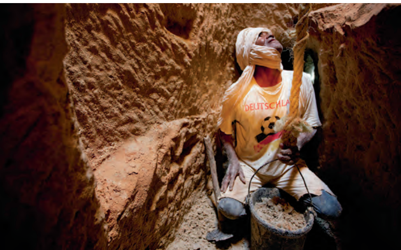
Near Akabli in south-central Algeria, an old qanat is being cleared, bucket by bucket, each one hauled 12 meters (38') to the surface.
